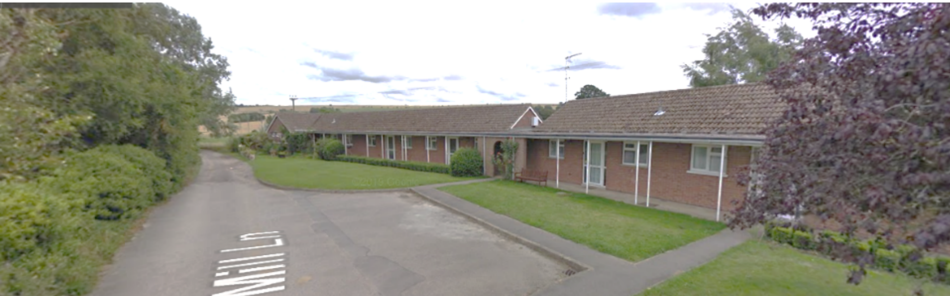
Terraces of bungalows at the east end of the Hedges House site
